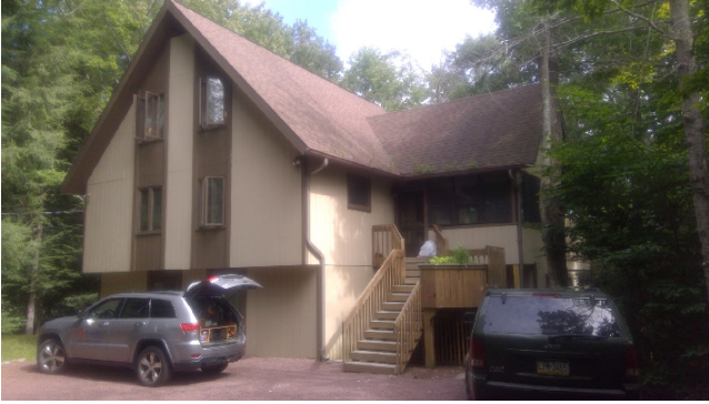
CP09 Front of house (PICTURE REQUIRED)
