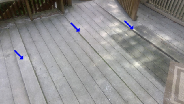
Lifting deck boards
