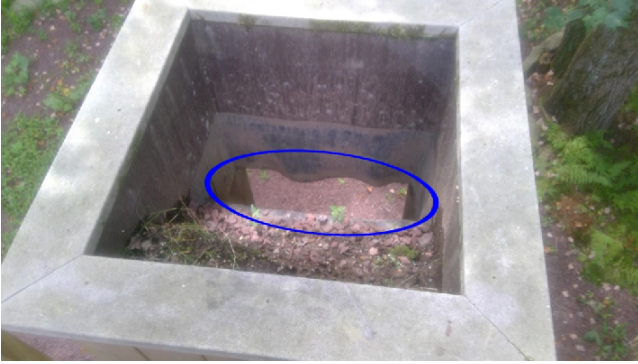
Planter rotted - hazard
