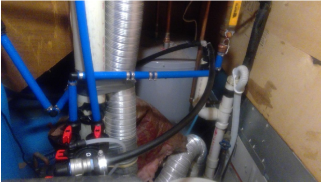
Limited view to components under stairs
